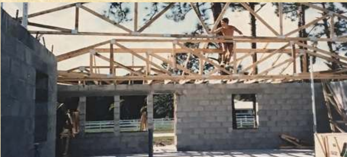
Setting the trusses on 5145 Grebel Lane
